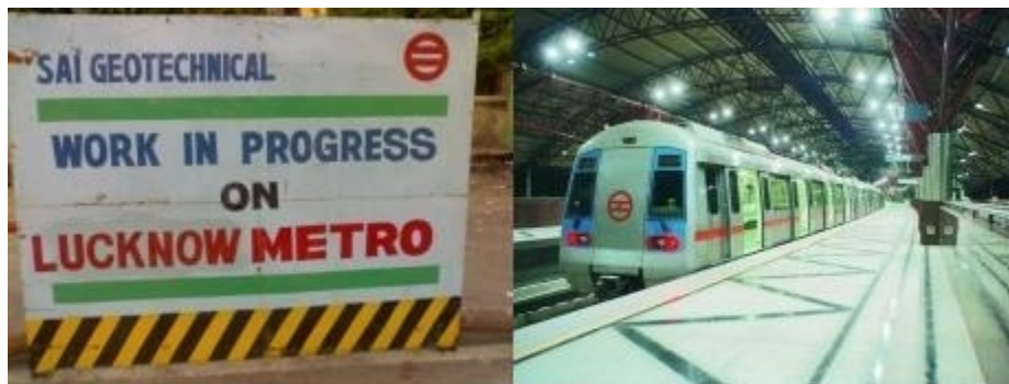
Lucknow Metro (WIP)
